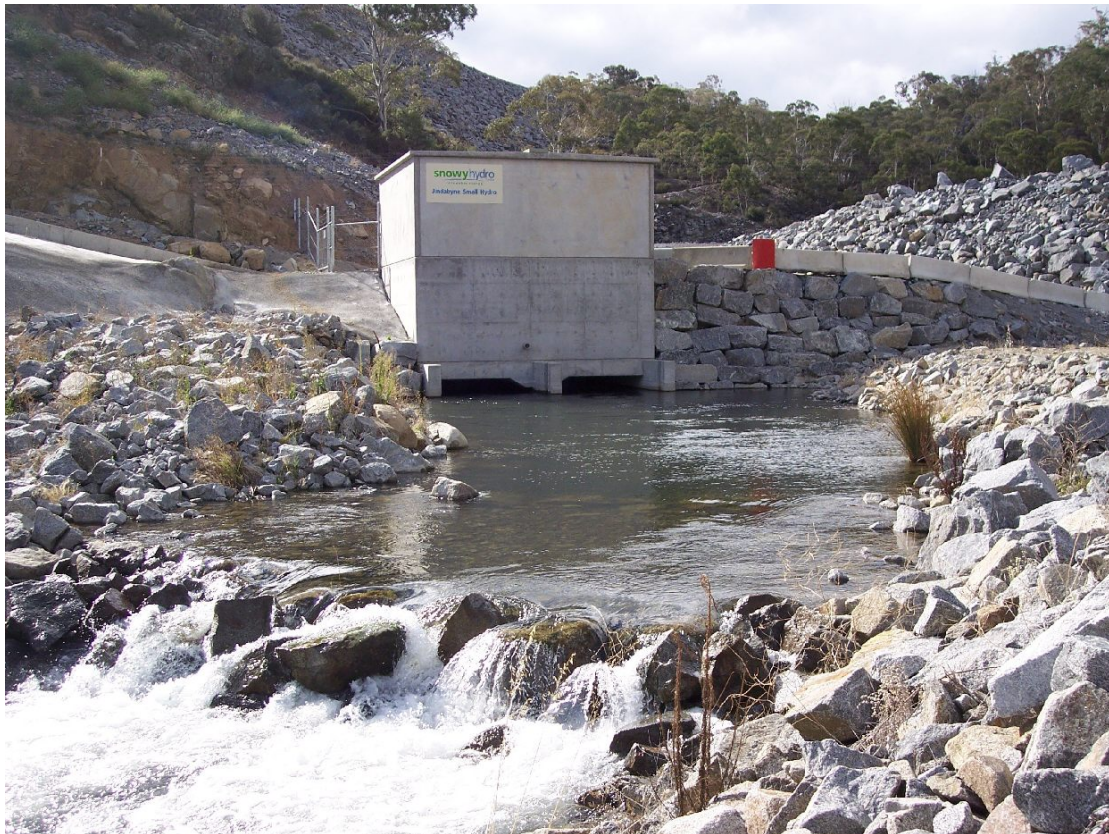
Total Snowy River Increased Flows - Jindabyne Dam mini hydro, April 2009
